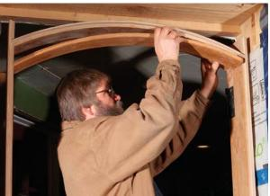
Fasten the jambs and install the stop. Once the side jambs are plumb and securely fastened with structural screws, the first layer of the two-layer stop is fastened to the head jamb with 1-in. screws. Then the side stops are coped around the head stop and screwed in place. The screw heads will be hidden by the second stop.
