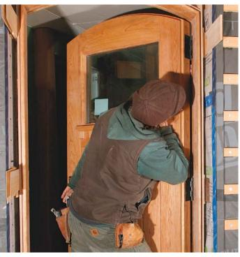
Hang the door. Once the first-layer stops are in place, the door is hung from its hinges and closed. The second stop is then held tight to the door and fastened through counterbored holes that will be filled with grain-matched cherry plugs later.
