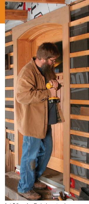
Install the casing. The jambs are taped to the house's water-resistive barrier with air-sealing tape, and then the casing is installed with screws. The screw holes are counterbored so they can be plugged later.
