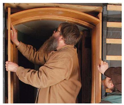
**Slip in the jamb extension.** Once both stop layers are in place, the assembled, three-sided jamb extension is fit to the main jamb with a rabbeted half-lap joint. A  $\frac{1}{4}$ -in. gap in the joint between the main jamb and the jamb extension allows for seasonal expansion. The gap is hidden by the stop.
