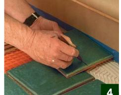
Mark cuts directly on the tile. There's no need for a tape measure when determining tile cuts. Just hold the piece above where it will be set, and mark one edge with a permanent marker.
