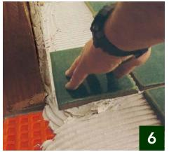
Mind the gap. The author aims for tiles to leave no more than a <sup>1</sup>/<sub>4</sub>-in. gap where they meet the wall. Any more than that, and you'll be wasting grout where it's not needed and taking a risk that the baseboard molding will not conceal the gap.
