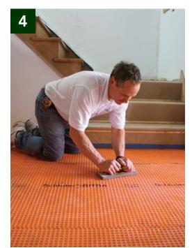
Bond it with pressure. To ensure a flat surface and a good bond with the thinset below, use a wooden mason's float to push out any bubbles. Start near the center of each piece, and work toward the edges. Use your body weight to lean into the float.
