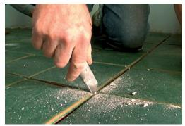
Clear the way for grout. The next day, after the thinset has hardened, use a utility knife to loosen any chunks of cement from between tiles, and then vacuum the whole floor.
