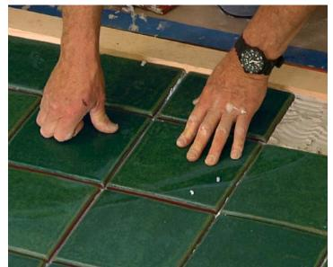
Use your eye, not tile spacers. Some tile installers use temporary spacers to ensure a consistent layout, but with handmade tiles like these, the variations in size and squareness of each piece make the spacers useless. Lay a small section, then adjust the tiles until the joints look even. When you get to doorways, use a level or a piece of wood as a guide to ensure a straight edge.
