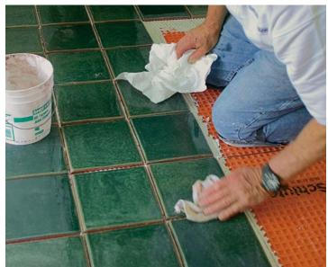
Clean and seal as you go. You won't be able to walk across the tile until the thinset has set up, so now is your chance to keep the surface neat. After laying tile in each section, wipe the surface with a tile sponge and as little water as possible, then apply a coat of sealer. The sealer is especially important when grouting stone tile or tile with a flat finish.
