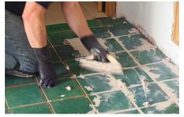
**Take the right angles of attack.** Spread the grout, and push it into the tile joints using a premium quality rubber float held at a 30° angle to the floor. After switching the float angle to 60°, scrape off the excess, being careful not to dig into the side of the joints.
