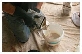
**Know the ABCs of mixing.** Combine part A and part B, the pouches of liquid epoxy, in a clean bucket. Mix the two liquids together with a margin trowel, and then add part C, the carton of colored filler.
