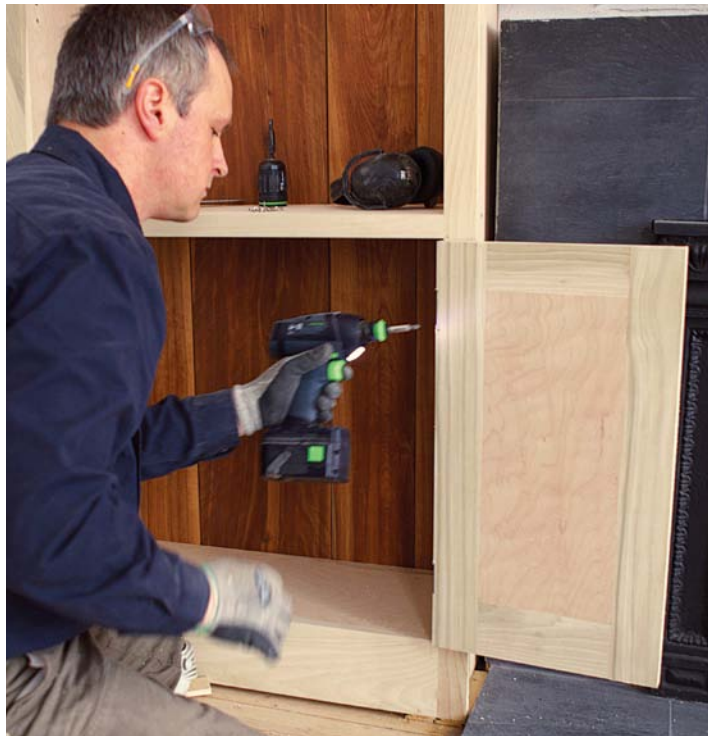
Hang and adjust in place. With the hinges in place on the cabinet doors, hold the doors in position while you transfer the hinge locations to the face frame. Attach the door, and tweak as needed for a perfect close.
