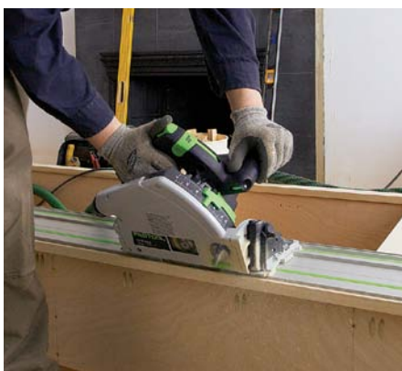
Trim the fat. Use a track saw to remove as much wood as possible without reaching the scribe line. Back-cutting at a 30^\circ bevel makes the hand-planing easier.
