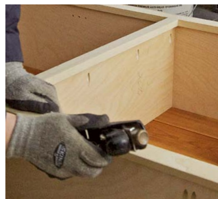
Finish with care. For a simple scribe, use a block plane to shave up to the line. Complicated scribes may need a jigsaw or an angle grinder with a sanding disk.
