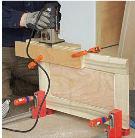
Site-made mortise jig. Plywood scraps are all that’s needed to make a custom hinge jig. A router with a flush-bearing bit rides the jig to cut the through mortise.
