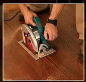
Divide the board. Using a circular saw set to the thickness of the flooring, make two parallel cuts along the length of each marked board, stopping shy of the end. If there are several boards in a row that will be removed, cut across their width to speed up the process.
