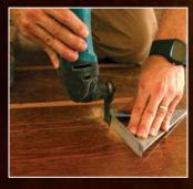
Make your own joints. When creating a new joint in the middle of an existing board, align a rafter square with the long side of the floorboard, and apply firm downward pressure to the square as you plunge the multitool along its edge.
