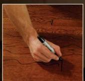
Mark a new layout. Use a marker to indicate which boards will be removed, and where any new butt joints will be added. Always carry the mark along the length of the board to avoid confusion when cutting, and stagger the joints by at least a foot or so.
