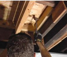
**Shim it flush.** Often the existing subfloor, usually  $^3$ /4 in. thick, won't match the thickness of modern plywood, which is often slightly thinner than  $^3$ /4 in. To make up for this discrepancy, glue and screw the new piece of plywood into place, but before the adhesive sets up, back off the screws and add shims below. When the top edge is flush, drive the screws home.
