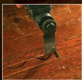
Plunge to finish the cut. The circular saw will leave a bit of uncut wood at the end of the board, which can be handled with an oscillating multitool. Plunge straight down until the blade hits the subfloor, being careful not to nick the adjoining board.
