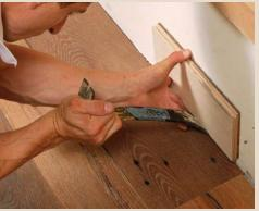
Squeeze it in. Use a flat bar to lever the last piece into place. A scrap of flooring used as a backer prevents the bar from damaging the drywall.
