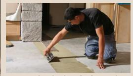
Start spreading the glue. After fitting and gluing the scribed areas in the hallway, use a <sup>3</sup>/<sub>16</sub>-in. V-notch trowel to spread the adhesive between the chalklines of the starter.
