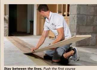
of flooring into the adhesive, and check to see that it's aligned with the chalkline. A couple of hammer taps help to set the pieces. As you fill in the rest of the starter, make sure the flooring isn't wandering over the line.
