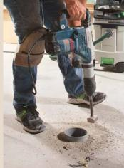
Flatten the high spots. Use a rotary hammer or angle grinder to grind down high spots, periodically checking progress with a straightedge. Afterward, sweep and vacuum the area.
