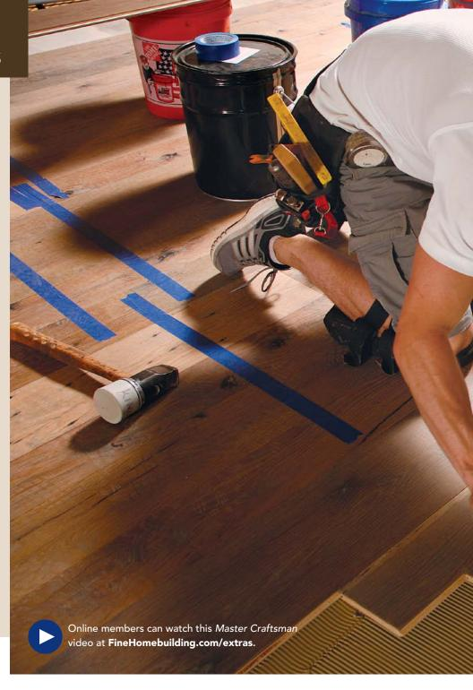
the starter row near the center of the room so that I can adjust in both directions. After measuring the space, I snap a chalkline along the long axis and check to see if it is parallel to each wall. A second line about 2 ft. from the first gives us the limits of the starter row.
