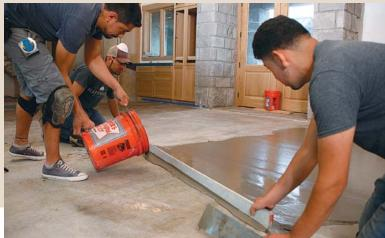
Make it flow. Mix the self-leveling compound, pour it onto a low area, and use a long straightedge as a screed to smooth its surface. Blend the edges into the slab with a trowel.
