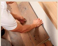
Rip and fit. After ripping the piece at the pencil line, test the fit, then spread the glue and drop the piece in. The width of the tongue on the scrap piece creates the <sup>3</sup>/16-in. gap at the wall.
