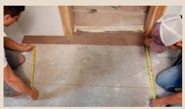
Dry-fit the first pieces. Because the flooring must fit under the cut door jambs and around jogs in the walls, dry-fit those pieces, then check to make sure that they are parallel to the chalkline.
