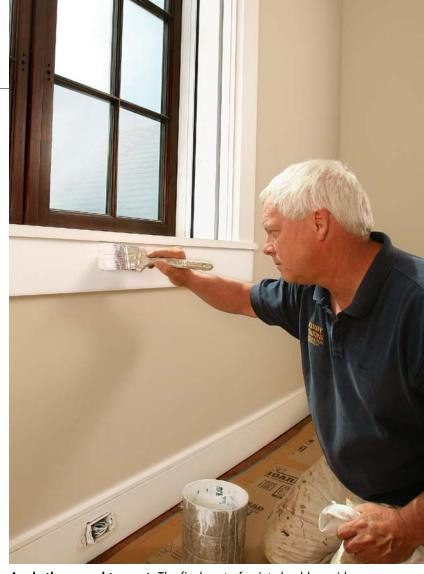
**Apply the second topcoat.** The final coat of paint should provide a perfect sheen and an extra layer of protection. After it has dried, check for missed spots and then clean the area, remove any masking, and reinstall the hardware.
