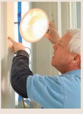
Shine a light. When a section is complete, use a strong light to make sure that all the imperfections are filled.
