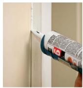
**Pull, don't push.** With the angled tube facing the crack, pull the tube along the seam as you squeeze out a consistent amount of caulk.
