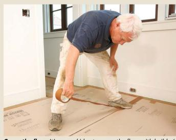
**Cover the floor.** It's a good idea to cover the floor with builder's paper to contain any embedded dirt. The author uses this quick method of footwork to apply tape to the paper.
