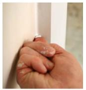
**Digital workflow.** Use a fingertip to smooth out the bead of caulk and to push it into the seam. Use a rag only to wipe off your finger, not the seam.
