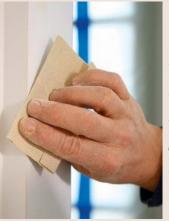
Don't forget the edges. Make all surfaces consistent by sanding the edges of trim pieces and the adjoining wall areas.
