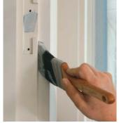
**Start from the edge.** To avoid buildup, brush first from the edges of the trim, making sure to hit the seam between the trim and the wall.
