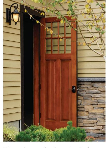
Highly exposed entrances on the south, west, and east sides of a home receive the harshest sunlight, making UV-resistance a necessity. Doors placed under eaves, porches, and other overhangs will be better protected. Most manufacturers of wood doors recommend that their doors be installed below an overhang that's at least half as deep as the distance between the sill and the eave. If you have less of an overhang, opt for a more durable door.
