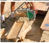
framing square. If the flanges are too wide for the cutting depth of my circular saw, I roll the saw over the edge of the I-joist to finish the cut (bottom photo).
