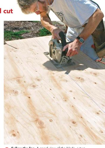
Follow the line. A good view of the blade, a twohanded grip, and a balanced stance ensure safety and accuracy.
