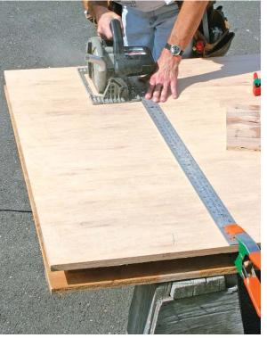
Make a guided cut. Running the saw's baseplate against a straightedge ensures a straight cut.
