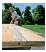
Mark the cutline. Support the panel on scrap lumber, and snap a line to mark where you need to cut.
