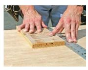
**Easy alignment.** Use an offset board to align the straightedge the correct distance from the cutline. The width of the board should equal the distance from the edge of your saw's baseplate to the blade.
