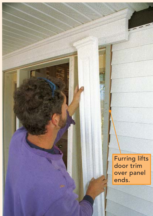
Door trim replaces J-channel. At a front door (right), a furring strip lifts the door trim enough to let siding panels tuck in behind.
