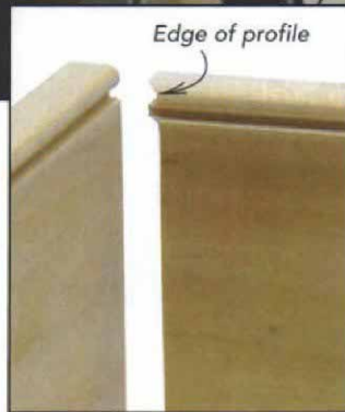
3 Cutting the profile. Following the edge of the exposed profile at a slight back bevel, the author uses a coping saw to finish cutting the profile.
